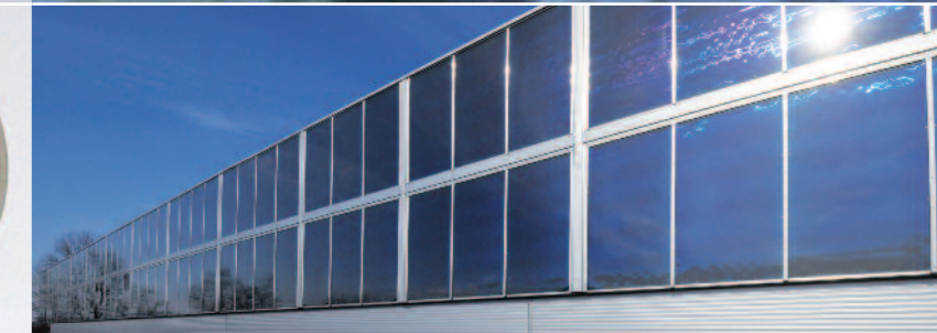
At Forstner Speichertechnik GmbH the office and the manufacturing are supplied only with renewable energies (a solar area of 252 m² supplies between 300 – 400 kWh/day even in winter).
